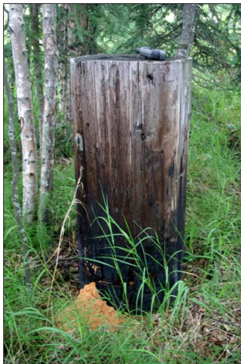
Figure 3. Base of creosoted pole in peat bog east of the Anchorage Police Headquarters south of Tudor Road.
